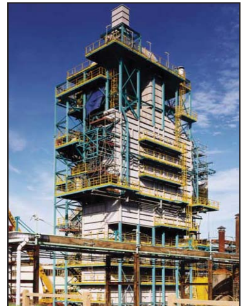
Ethylene Cracker Unit
